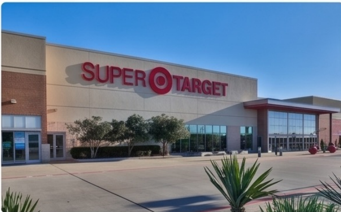
Lewisville Towne Crossing DISTANCE 6.95 MILES Total Retail Space >238,430 SF
